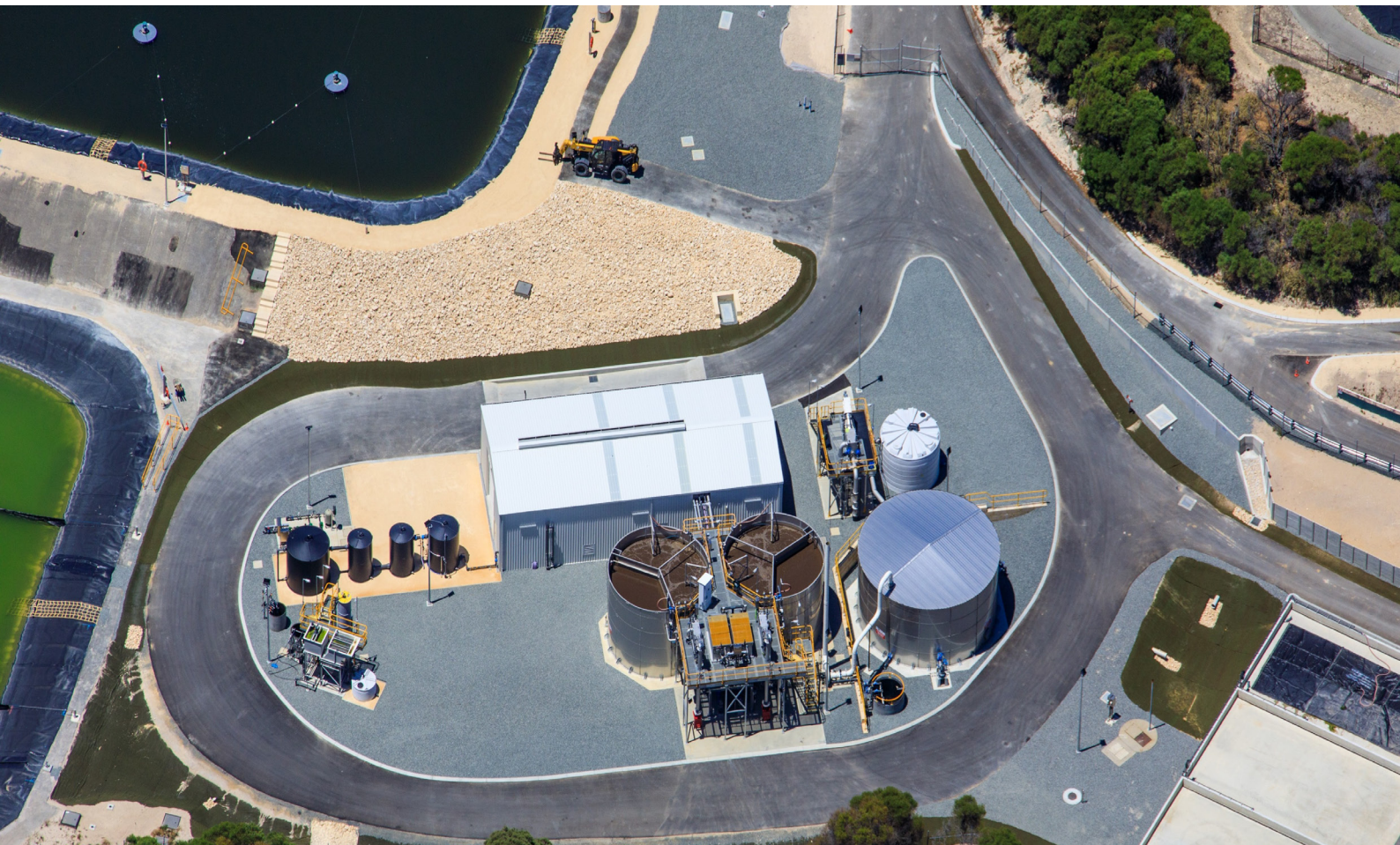
HMAS Stirling WWTP, Providing an essential service for the defense base upgrade
